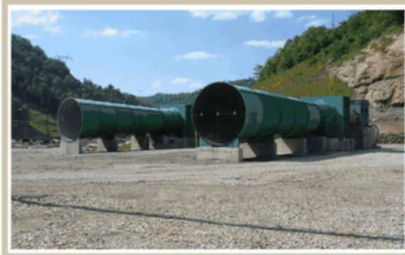
(return shaft fan installation)
