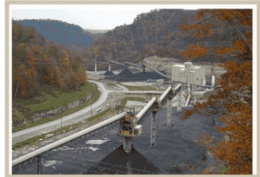
(raw and clean coal storage)
